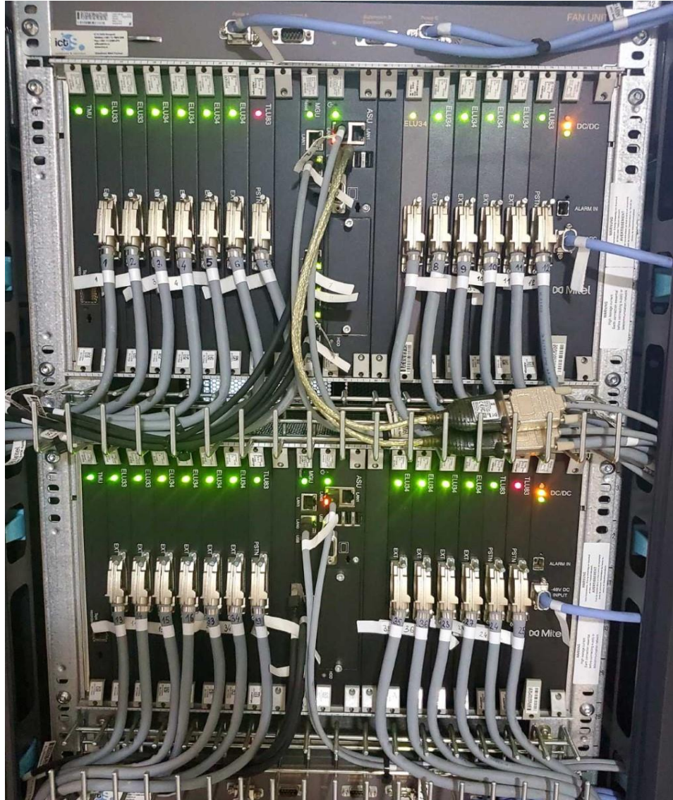
Figure 2 – Appearance of a modern, IP-oriented, transit PINX type MX-ONE Service Node 6.0 at a telecommunications center in the Air Force (Svrzić, 2019)
